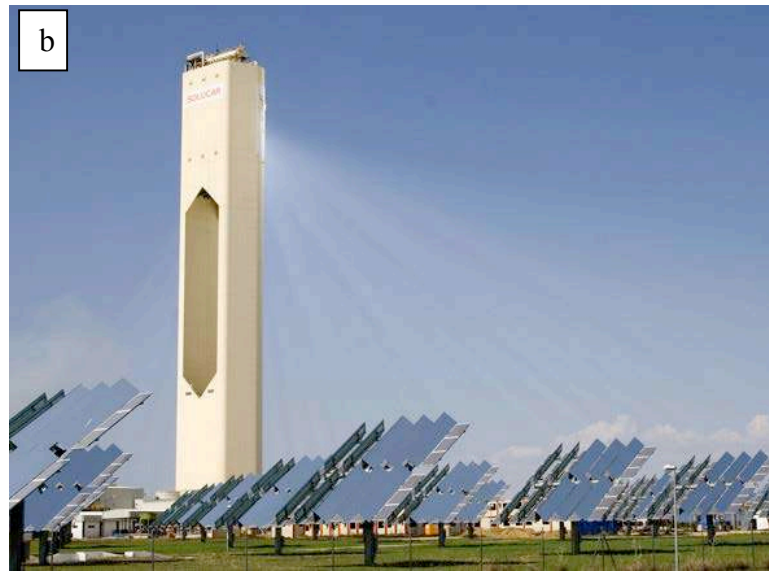
Figure 5.6: a) Rooftop Solar Installations on Douglas Hall at the University of Illinois at Chicago has no effect on land resources, while producing electricity with zero emissions. Source: Office of Sustainability. b) Solucar PS10 solar power tower in Andalusia, Spain, is a solar thermal power plant that generates electricity commercially. (Photo by Afloresm Solucar PS10 CC BY 2.0)
