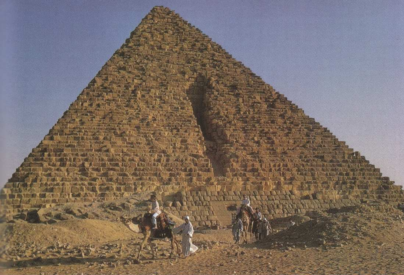
Menkaure's pyramid, with the great gash in its north face made by Othman in AD 1196. Below it, some intact granite casing is visible.
