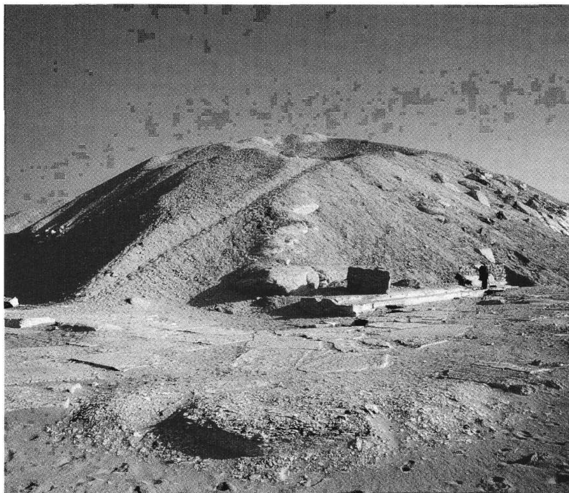
The pyramid of Senwosret I is now only a low mound, just 23 m (75 ft) high. Here, the end of one wall of the internal framework skeleton is visible through the debris.
