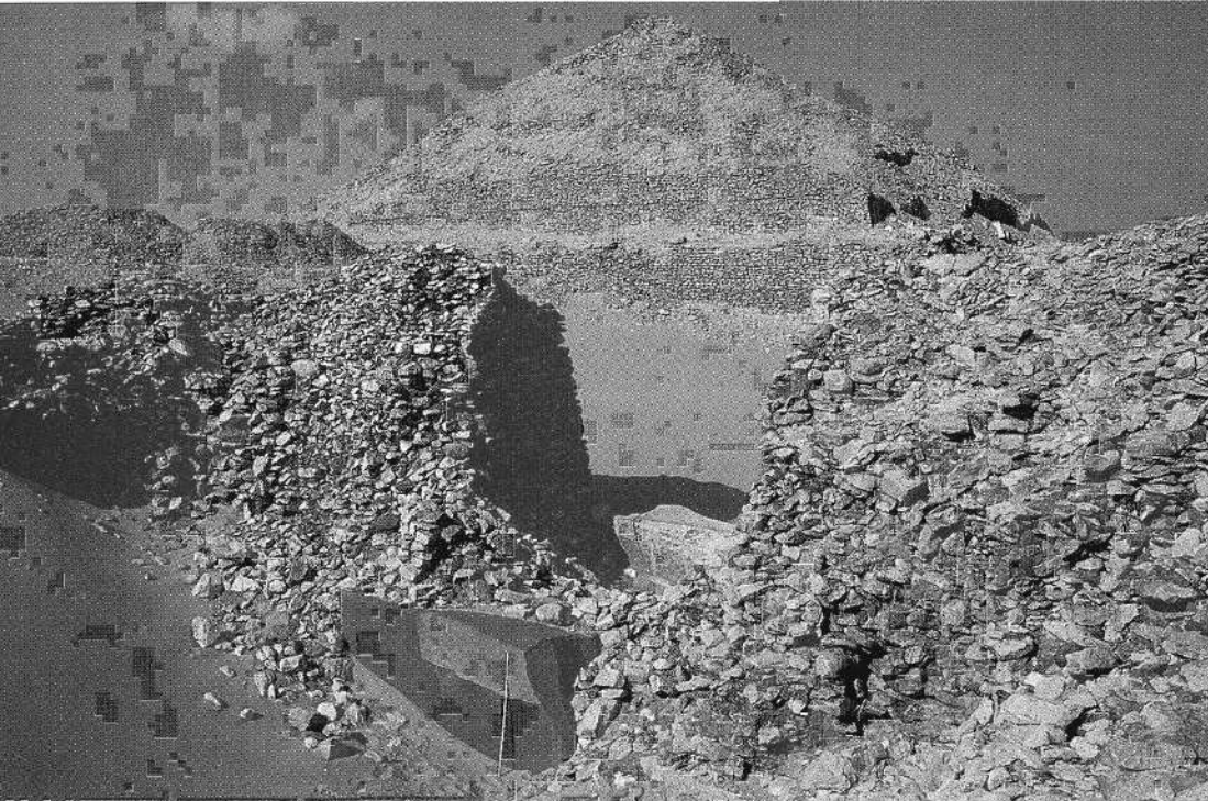
(Above left) The pyramid of Pepi II looking northwest over the ruins of Wadjebten's pyramid, with packed stone and clay core walls typical of the complex.
